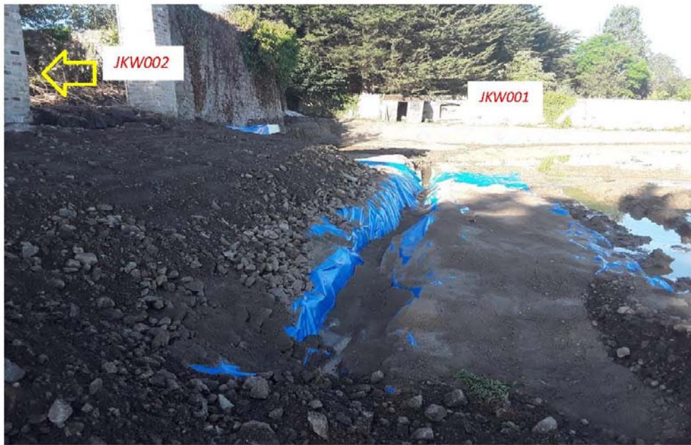
Image of Geo- Textile Root Barrier between JKW001 & JKW002.
