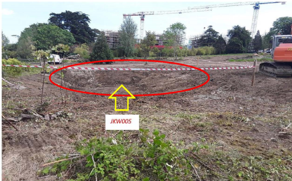
Image of JKW005 excavation. No JKW present in September 2019 or May 2020.
